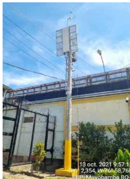
Fig. 8. Blocker and hardware to reduce propagation
